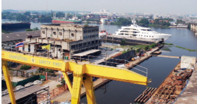
The new refit facility in Bangkok, Thailand
